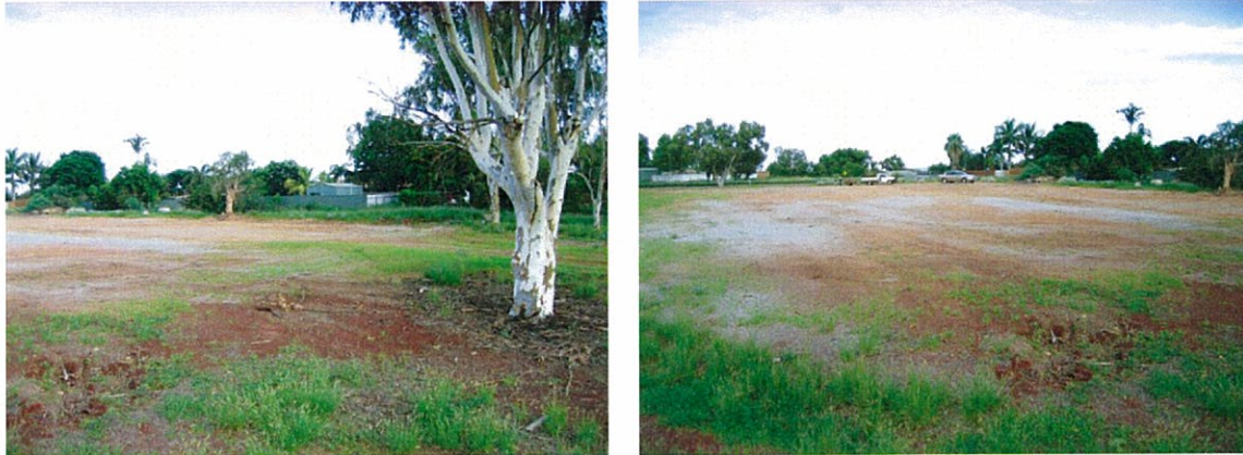
Figure 1 Photos of Block D indicating the shallow open drain and the flat topography across the site.
